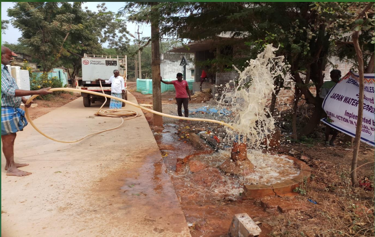
Cleaning of Bore water using a water compressor equipment
