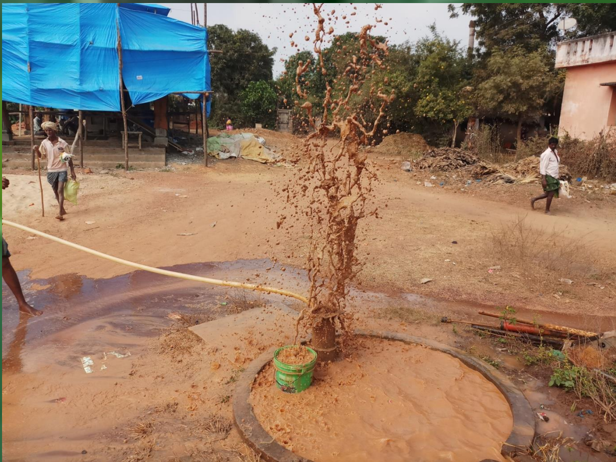
Removing of mud that is accumulated in the bore well
